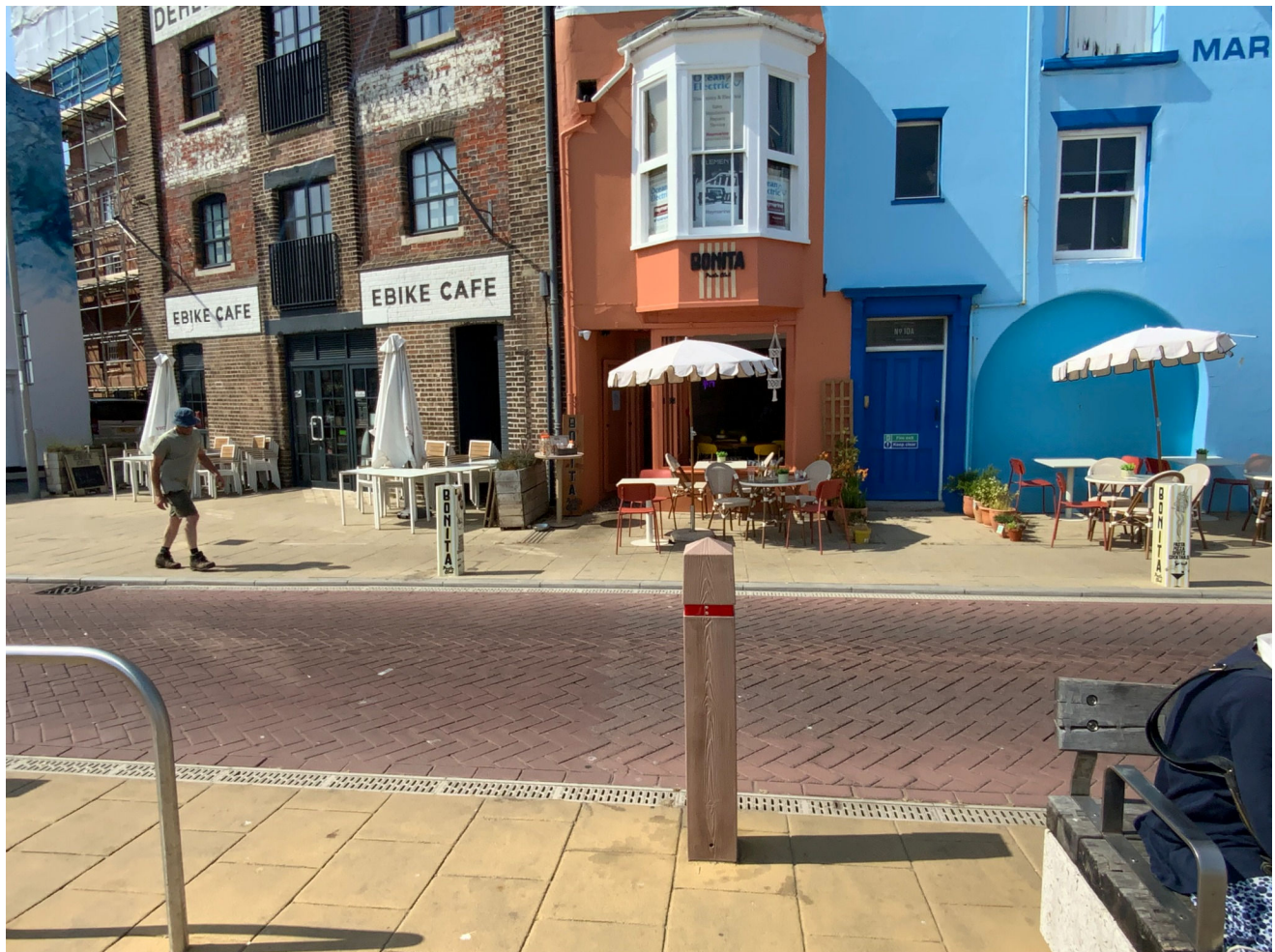
Figure G1 - Harbour frontage and local setting
